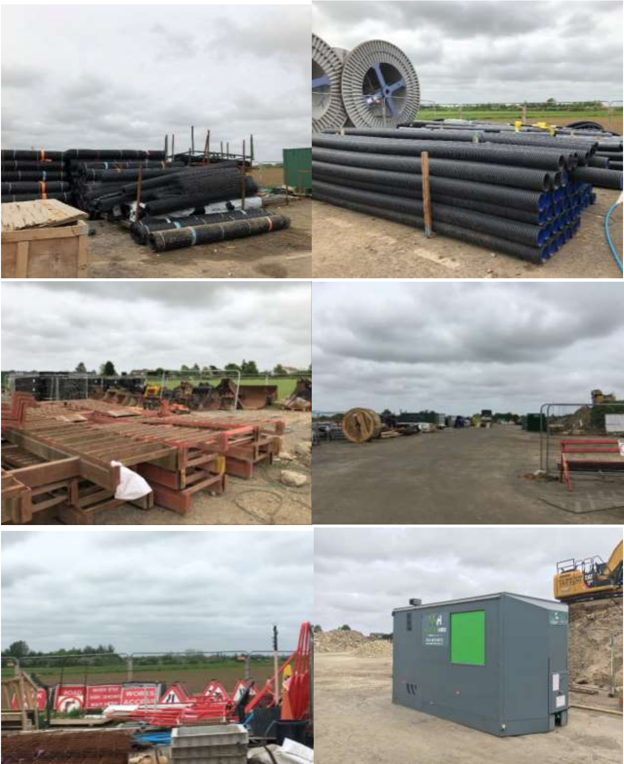
Figure 3.1: Images from Hornsea Project One Offshore Wind Farm Main Construction Compound (top left: storage of herras fencing); middle left: rumble strips; bottom left: signage; top right: ducting and cable drums and middle right: general storage; bottom right: portable welfare facility)
